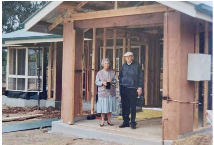
Pic: Marguerite & Thomas in front of the construction of their Villa
